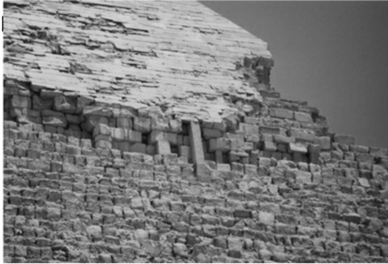
*Detail of the section of the Pyramid of Khafre where the Arabs abandoned their work in removing the cover stones. It reveals the extraordinary precision involved in the building work of this and other pyramids.*
