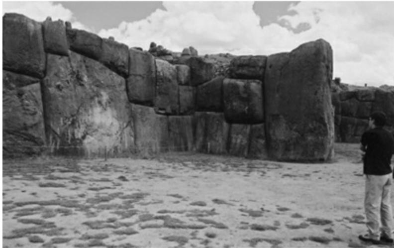
*The site of Sacsayhuaman, located just above Cuzco, displays some of the largest and most extraordinary stones. The stones have several differently shaped sides, which somehow all fit perfectly together. This technique was necessary because of the severe earthquakes prevalent in the region. The Inca's construction technique has proven to withstand these quakes when no other buildings did.*
